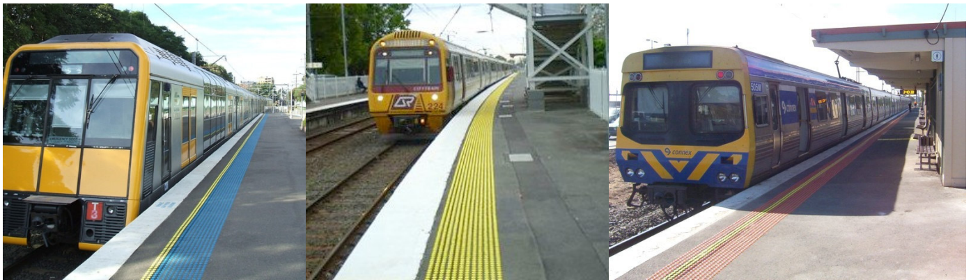
Installation of single stud, full polyurethane tactile indicators
