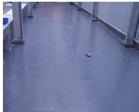
Waterproofed anti-slip concrete floor
