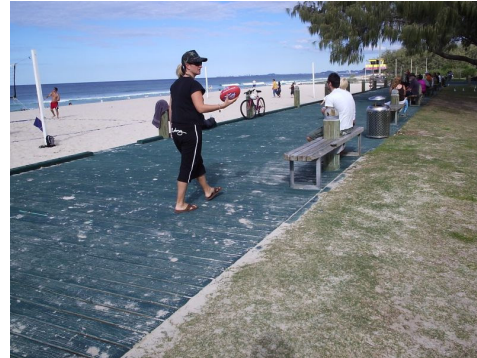
Anti slip coated timber boardwalk
